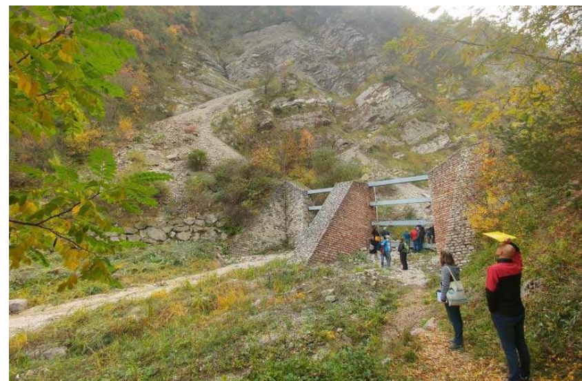
Outdoor module: Ravina and Gola stream (TN)
